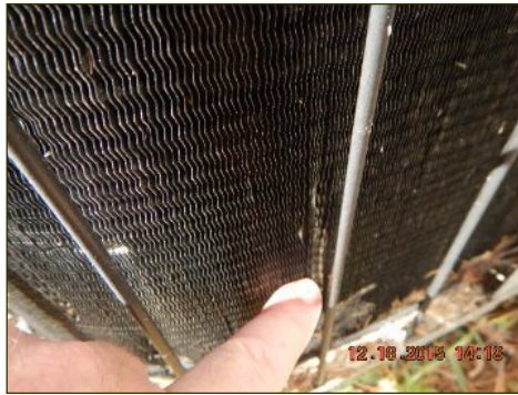
Fin damage observed on heat pump
