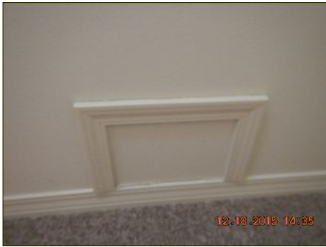
Motor access sealed
