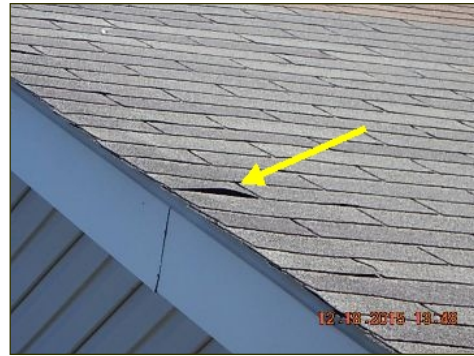
Shingles should be sealed
