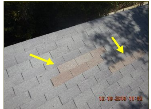
Different colored shingles suggest Prior repairs
