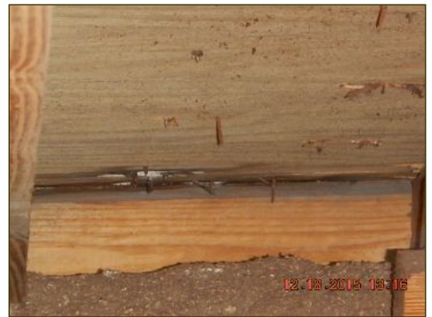
Rot/deterioration noted at north side of home
