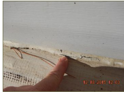
Sealant needed at chimney
