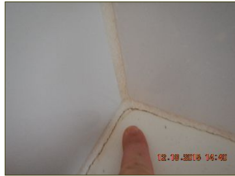
Caulking maintenance needed at whirlpool tub
