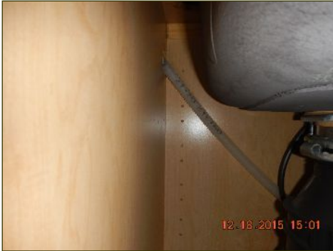
No high loop to dishwasher drain hose
