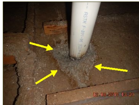
Insulation stained below flashing
