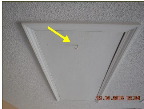
Access missing pull down string
