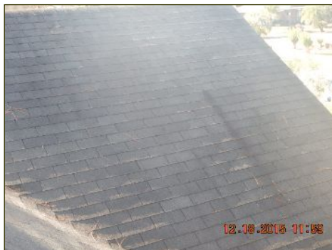
Staining noted on roof covering
