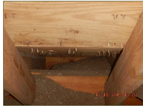
Soffit vents congested in various locations
