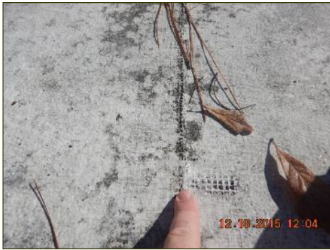
Prior repairs observed on porch roof
