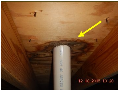
Staining below plumbing vent flashings
