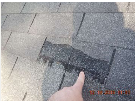
Damaged shingle at west side of home
