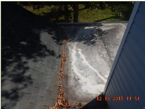
Recommend removing debris from roof
