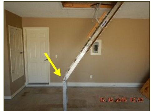
Attic stairs not folding properly
