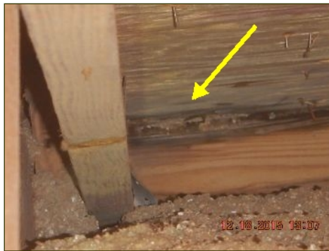
Rot/Deterioration noted by flat roof-chimney
