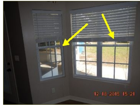
Windows should be adjusted so they remain upright
