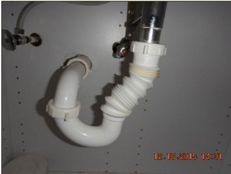
Corrugated drain pipe
