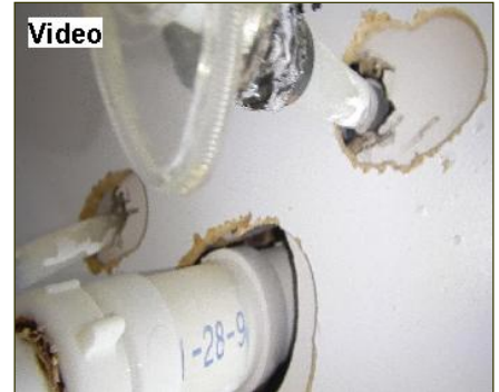
Click to watch video of leaking supply valve
